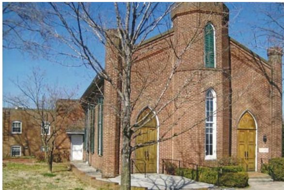
Hendersonville 1 st Presbyterian Church
