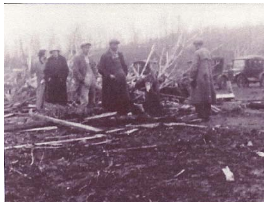
The wreckage of the Holmes' house
