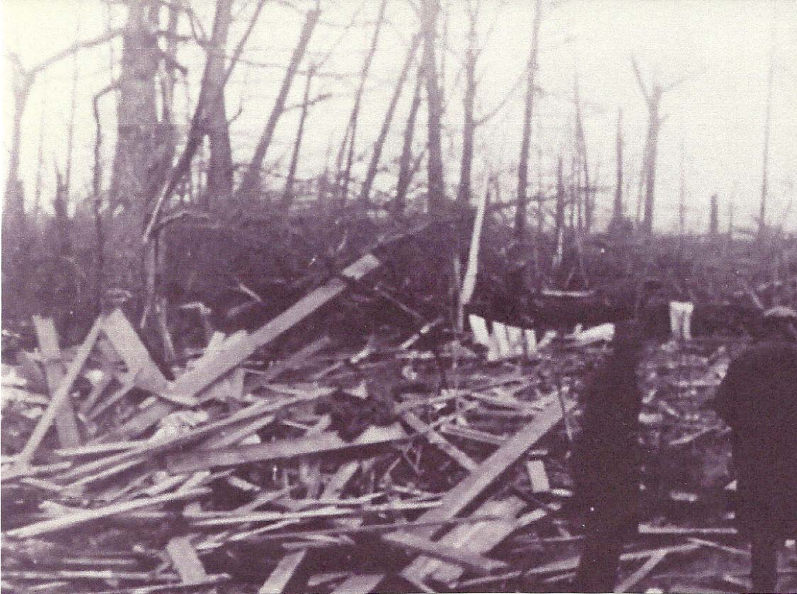
In this archives photo, neighbors are shown at the wreckage of the Allison house where nine perished in 1925
